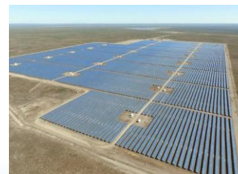
BYD Solar Power
